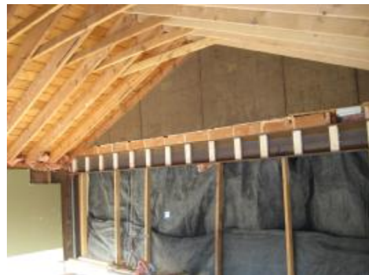
A new steel header supports second floor loads.
